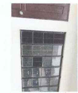
INSTALLATION OF NEW GLASS PANEL, 0.35m x 0.3m
