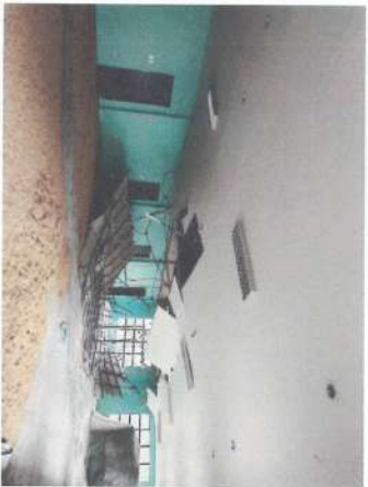
AREA FOR CEILING REPLACEMENT, INSTALLATION OF NEW FIBER CEMENT BOARD
