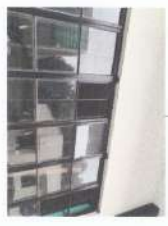
INSTALLATION OF NEW GLASS PANEL, 0.35m x 0.3m
