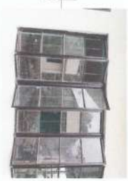
INSTALLATION OF NEW GLASS PANEL, 0.35m x 0.3m
